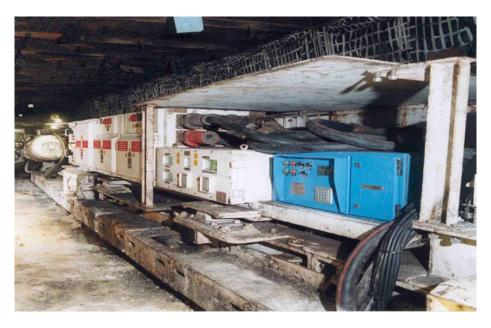
The PLCs control Machinery including the coal-face coal shearing machines, ventilation, and conveyors. The coal face at Daw Mill is currently 10km from the control room; therefore communication has to be fast and effective - fibre optic Intrinsically Safe Ethernet is being used throughout the mine.
