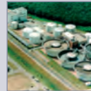
WASTE WATER TREATMENT PLANT
