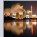
COAL FIRED POWER PLANT
