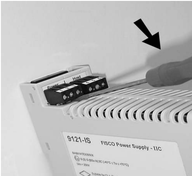
Figure 14 - Disconnection of FISCO power supply terminal block
